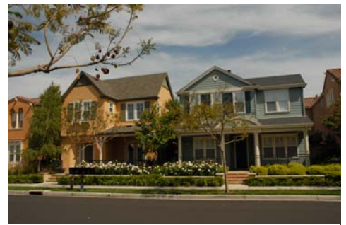
Respondents gave high ratings to this street elevation of small-lot single-family housing in Santa Clara.
