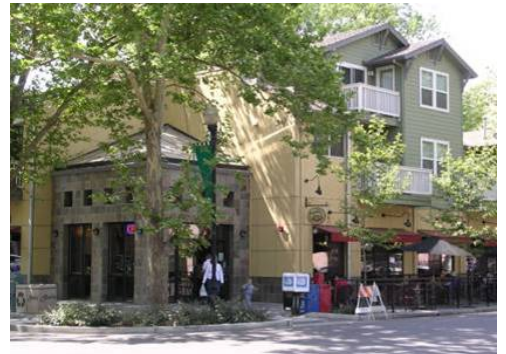
The two most well-received higher-density developments were, again very different from one another: Sierra Oaks, a large development in Turlock with a unified appearance (left), and a small mixed-use project in Davis.
