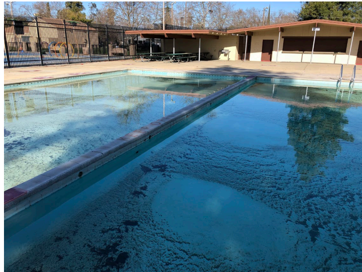
Wall Within Swimming Pool
