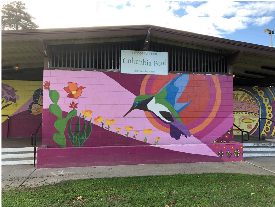
Entrance to Columbia Swimming Pool
